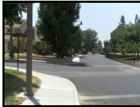
Duarte Golf Course – Canyon Park LF – SWCP Grant to correct Drainage & Erosion/RPs hired consultant/contractor to remedy LFG Violation
