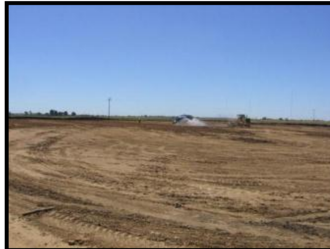
Franklin Field Burn Dump - Capping & Grading (SWCP Grant)
